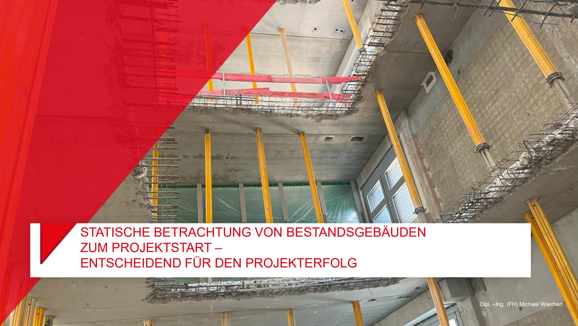
The image shows the interior of a building under renovation. Numerous yellow steel columns are visible, supporting the ceiling. A large red safety netting or tarp is draped over the left side of the frame. In the background, there are concrete walls, a window with white blinds, and exposed rebar structures. The overall scene is one of active construction.
