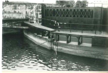
Doppeltes Stemmtor (Fluttor, Ebbetor)
