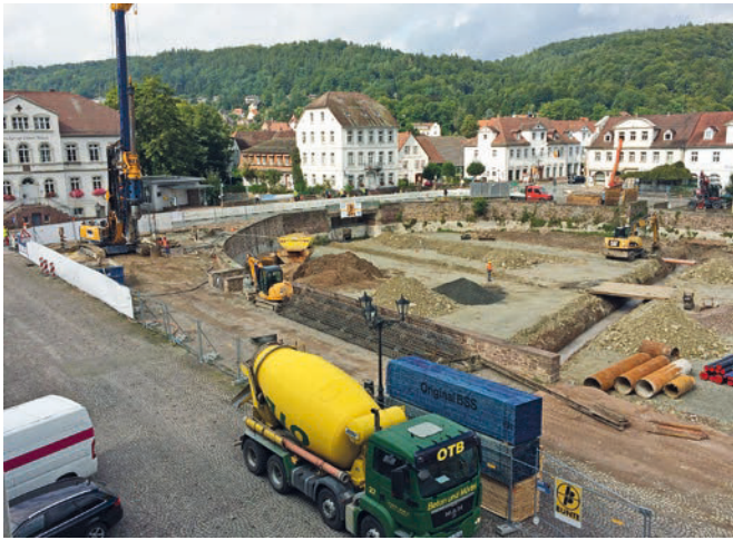
Bild 10 Baustelle (Stand 09/2017) Building site (status 09/2017)
